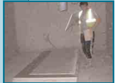
Plasterboard placed on the floor, requiring the operative to stoop to pick it up or trim it to size.
