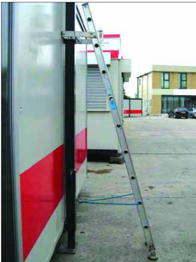
Figure 4 Specially designed ladder, fitted onto the cabin.
