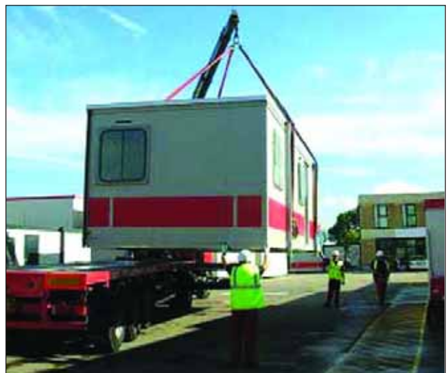
Figure 2 A successful lift with slings in place
