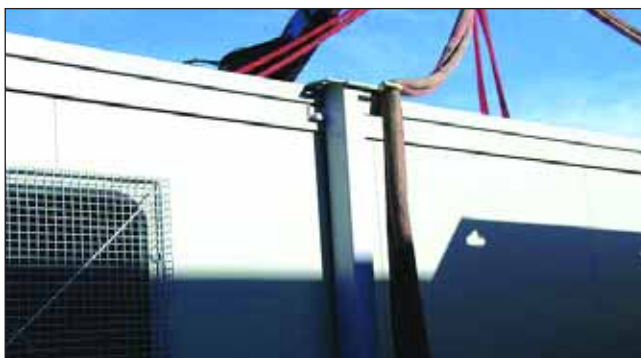
Figure 1 Brackets, retrofitted to the bottom and top of each cabin jackleg.
