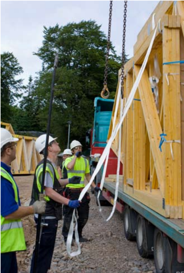
Figure 3 Slings accessible from the ground
