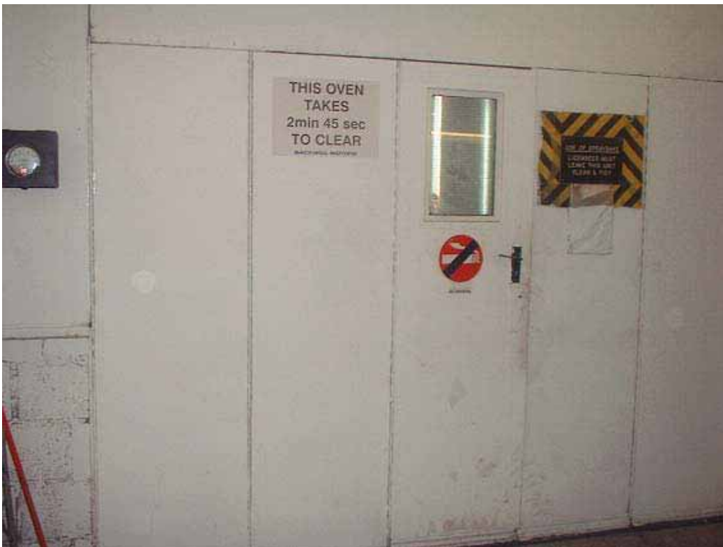
Photograph 2: Clearance time displayed on booth doors
